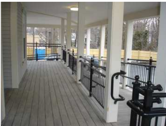
New Accessible Entry / Porch
