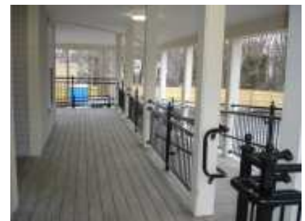
196 Federal Street, Greenfield New accessible entry / porch
