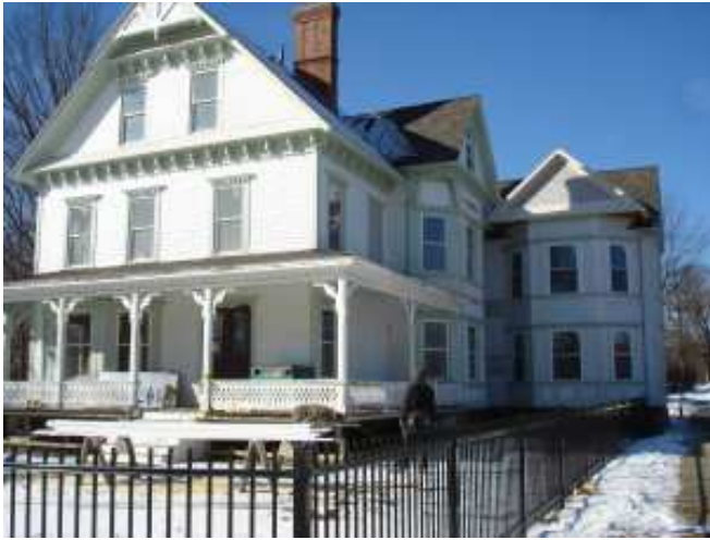
After Addition (progress photo)
