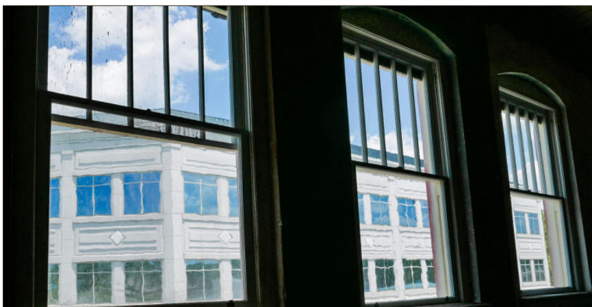
Above: Council member Bill Grant, left, looks at exposed ceilings in the basement level of an interior tour of the Jones Building. Below: Jones Building original windows were taken offsite for lead paint removal and reinstalled. / Staff-Margaret Waage
